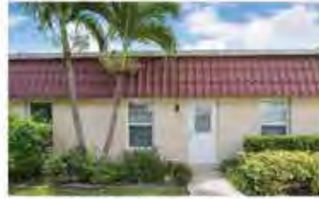
www.246DownEastLaneA.com Spacious and flawlessly updated villa in Covered Bridge!
