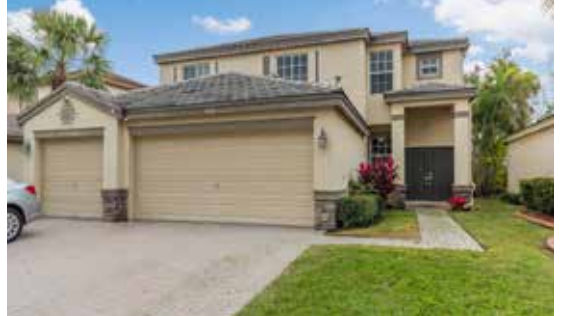
5816 Saddle Trail Lane great home in Thoroughbred Lake Estates
